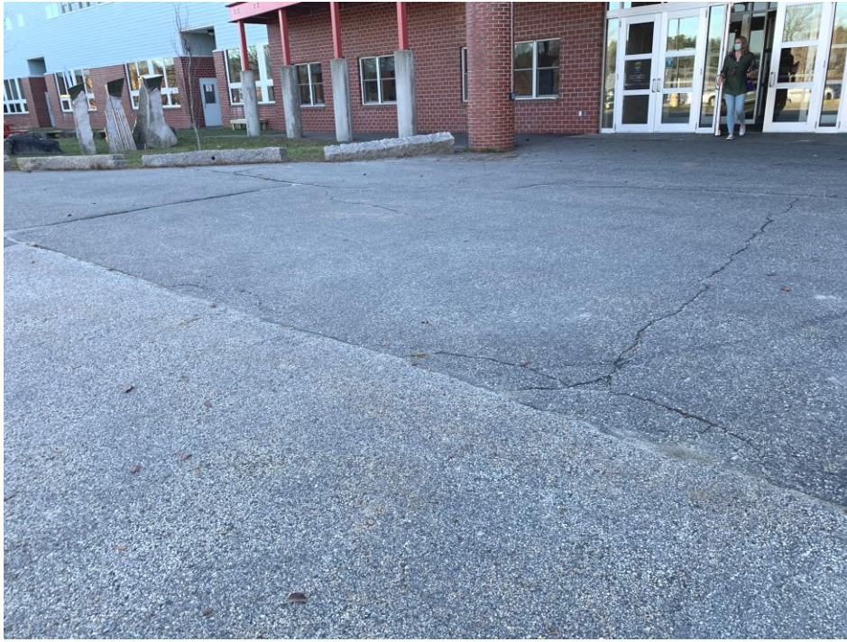
Mt. Ararat Middle School main entrance plaza
