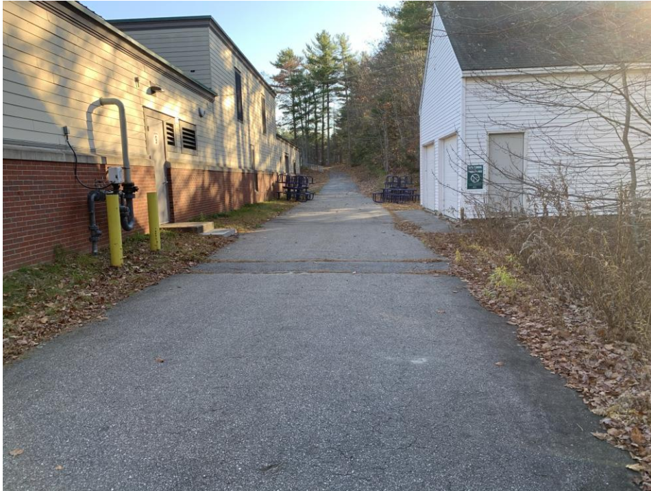
Woodside Elementary School service drive along back of school
