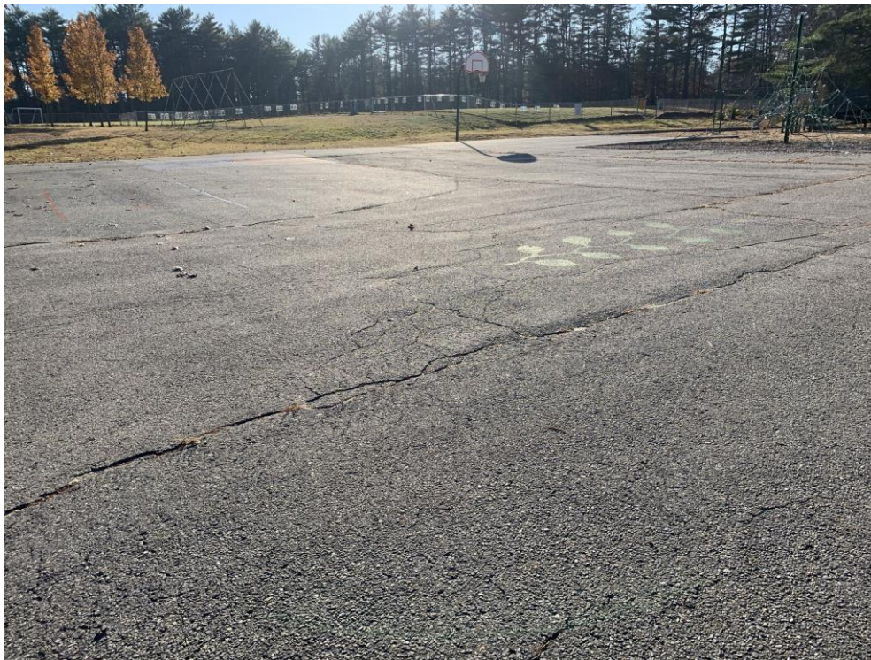
Woodside Elementary School paved playground
