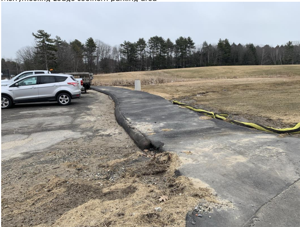
Merrymeeting Lodge southern parking area showing new sidewalk
