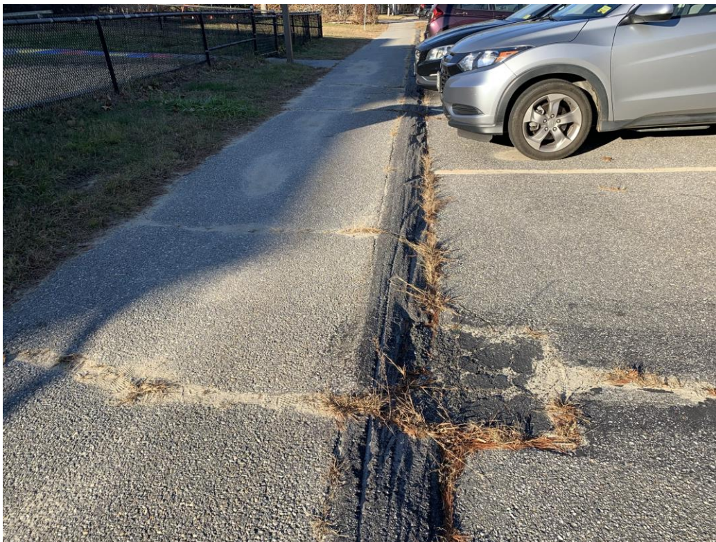
Woodside Elementary School southeast parking area
