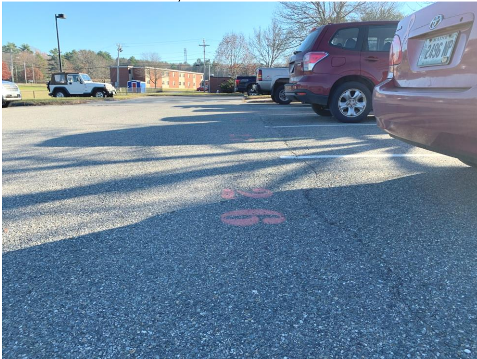
Mt. Ararat Middle School East Parking Area is in fair condition
