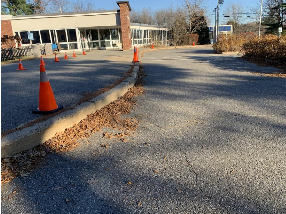
Williams-Cone School main entry plaza & bus drop-off
