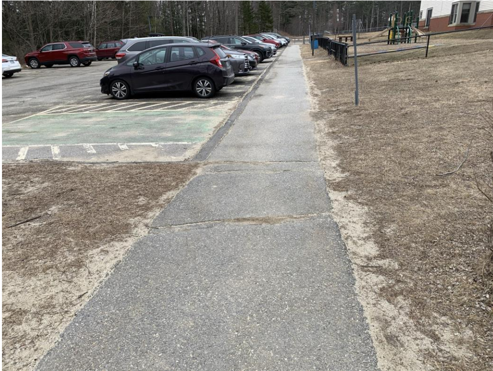
Sidewalk bordering the southern parking area
