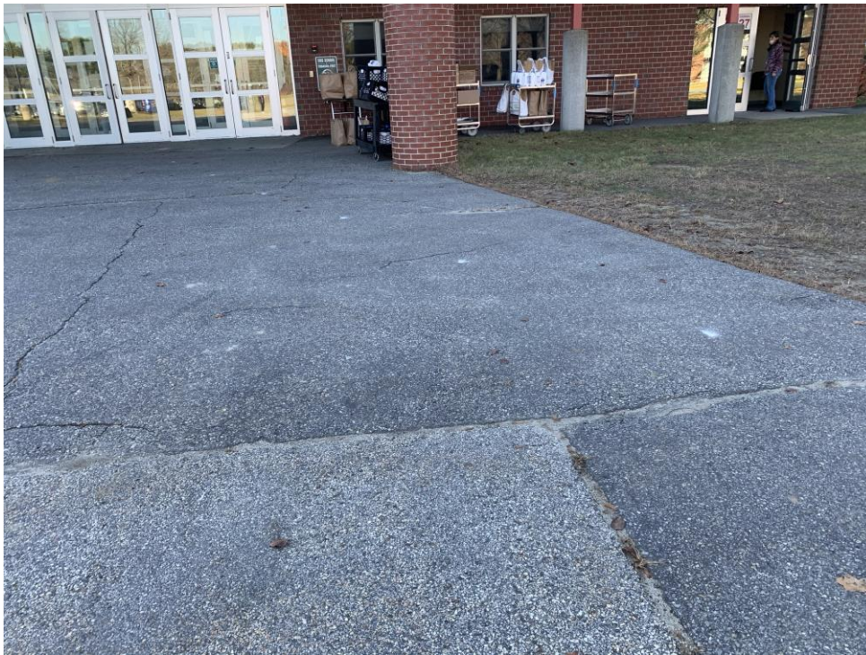
Mt. Ararat Middle School main entrance plaza
