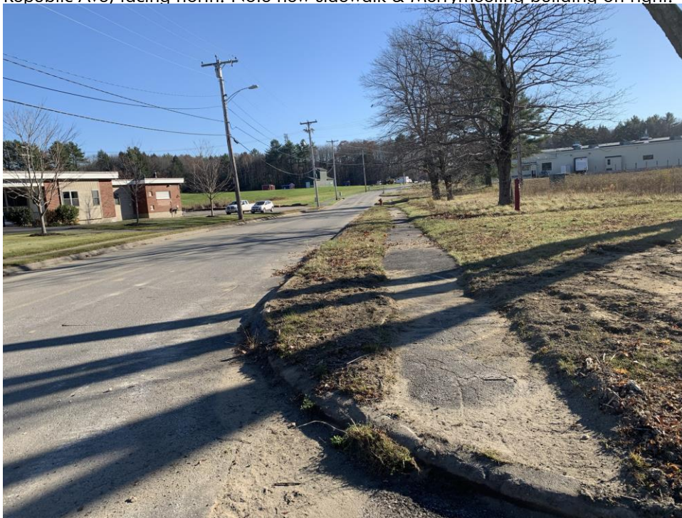
Republic Ave, facing south, showing abandoned sidewalk.
