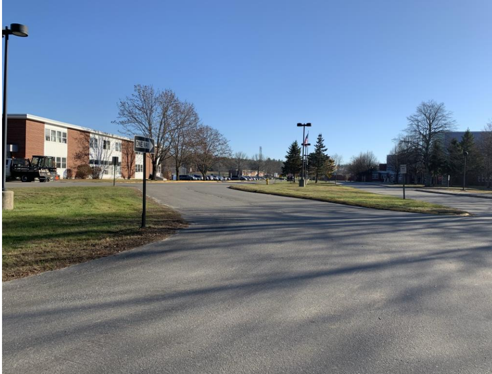
Mt. Ararat Middle School Republic Ave facing south from cul-de-sac with bus lane on right
