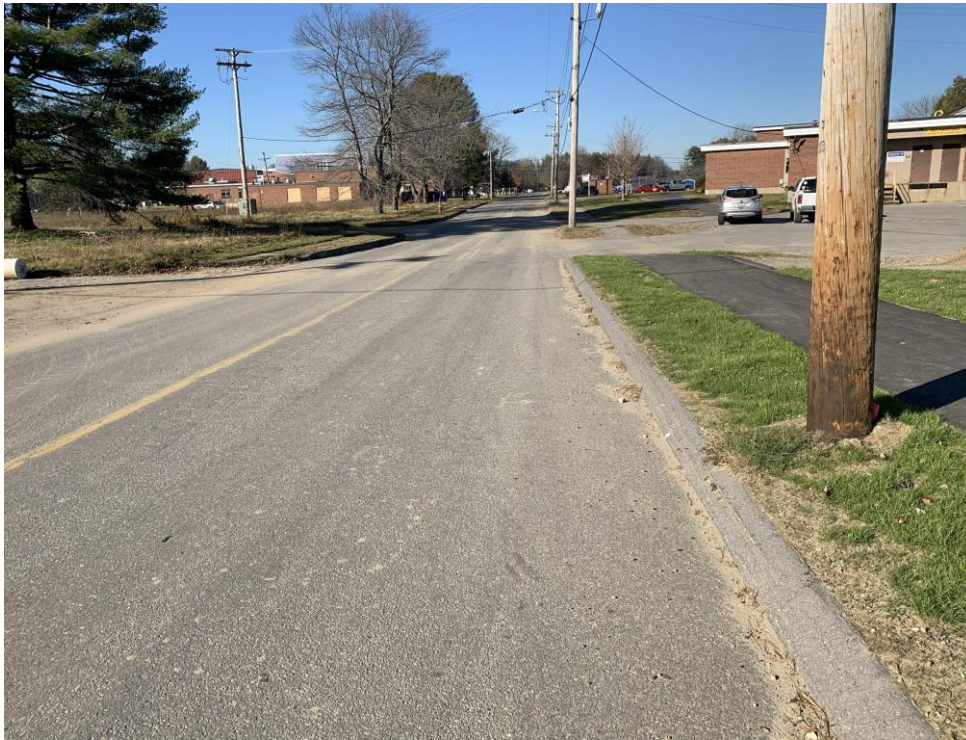
Republic Ave, facing north. Note new sidewalk & Merrymeeting building on right.
