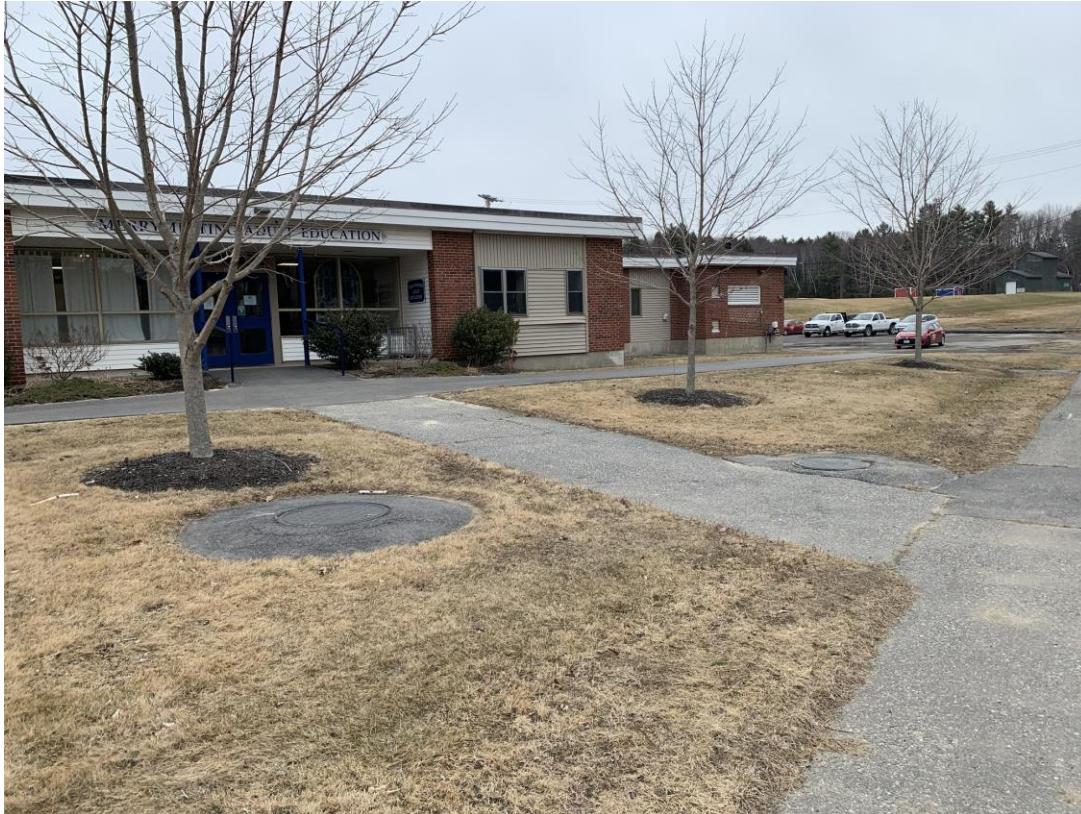
Merrymeeting Lodge connecting sidewalk between the new sidewalk and Republic Ave.
