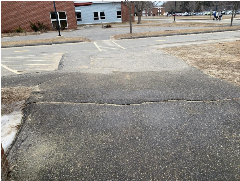
MSAD Office walkway at main entrance
