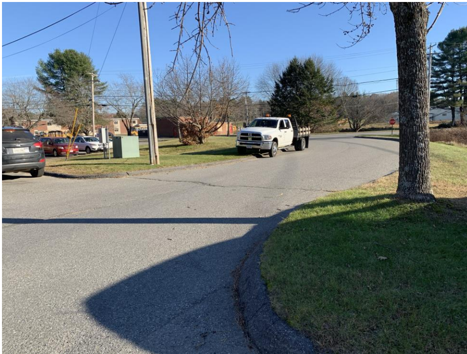
The MSAD office main drive looking back out to Canam Drive
