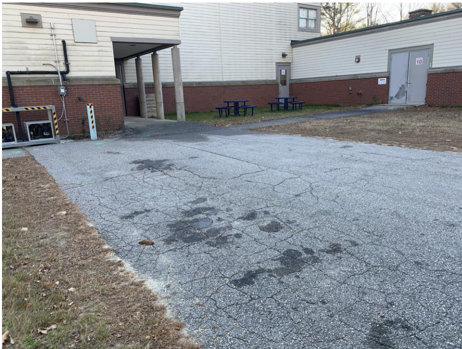
Woodside Elementary School service drive at loading area
