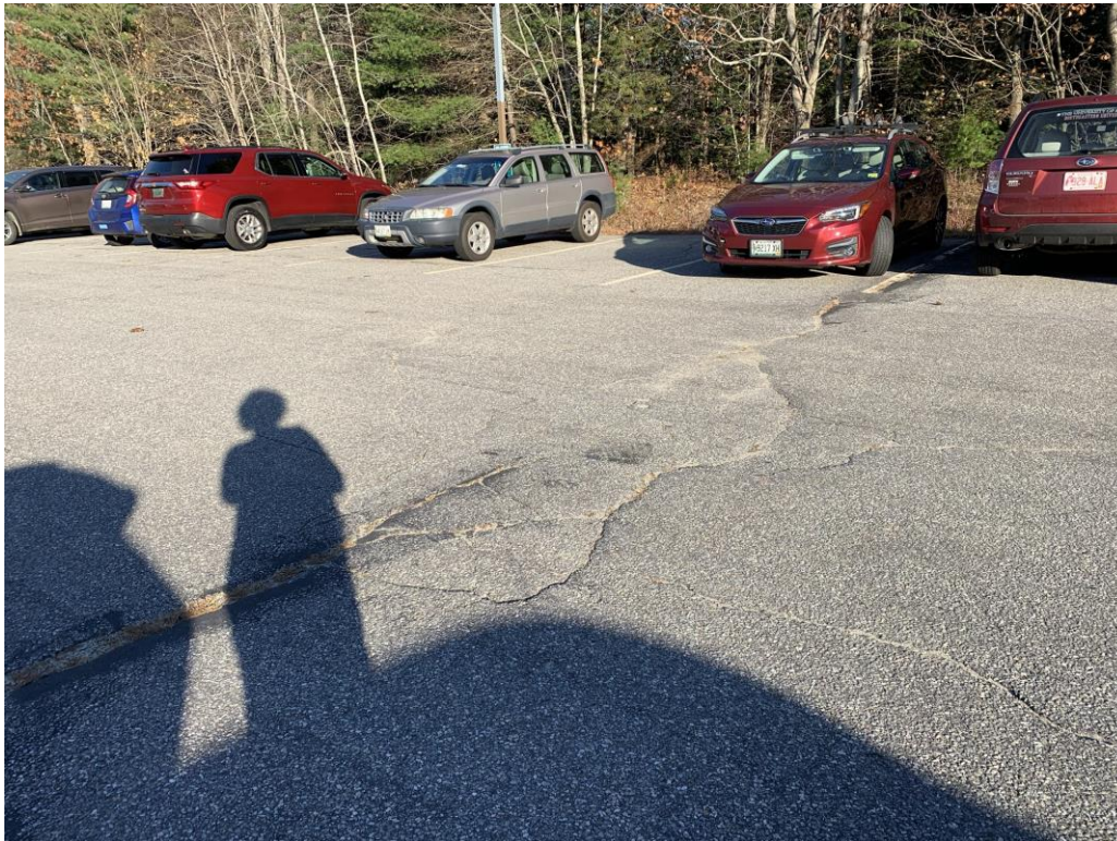
Woodside Elementary School southeast parking area
