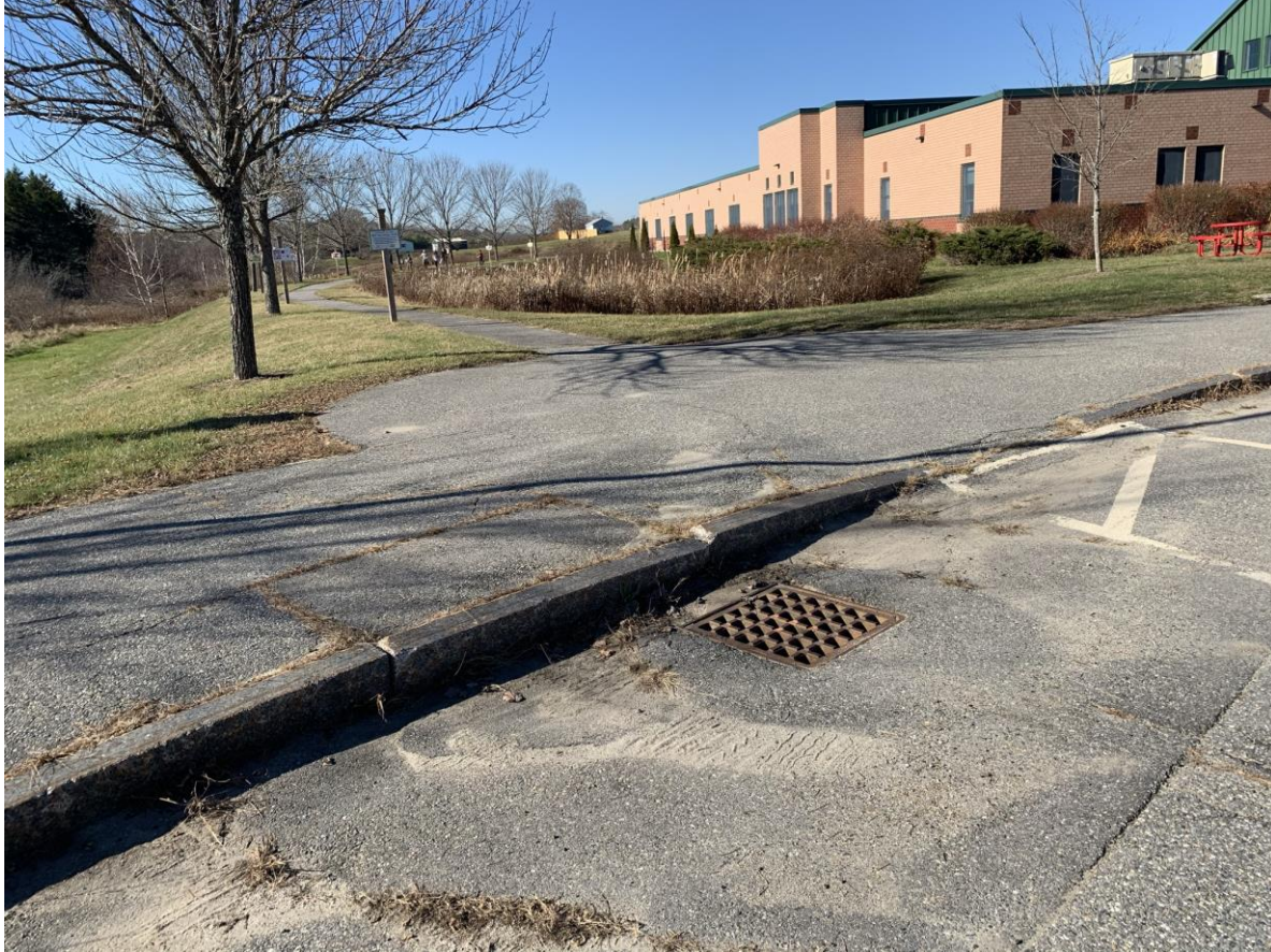
Bowdoin Central School Interpretive trail walkway
